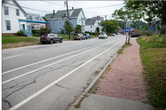
Congress Street looking east near Frederic Street showing aging brick sidewalk and bike lane dangerously close to active travel lane
