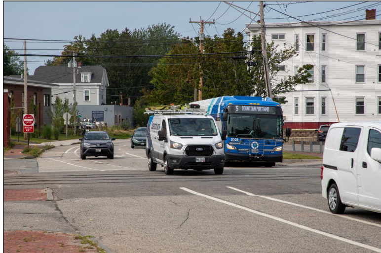
Congress Street (one way) looking west at the CSX/Amtrak railroad crossing
